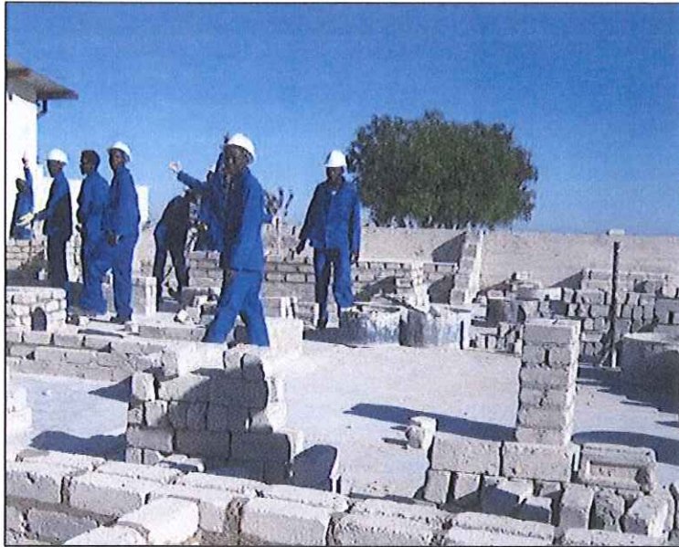
Some of the NIMT trainees in action with bricklaying.
